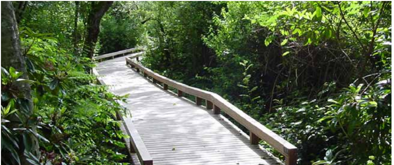
Luther Burbank Park north wetland boardwalk
